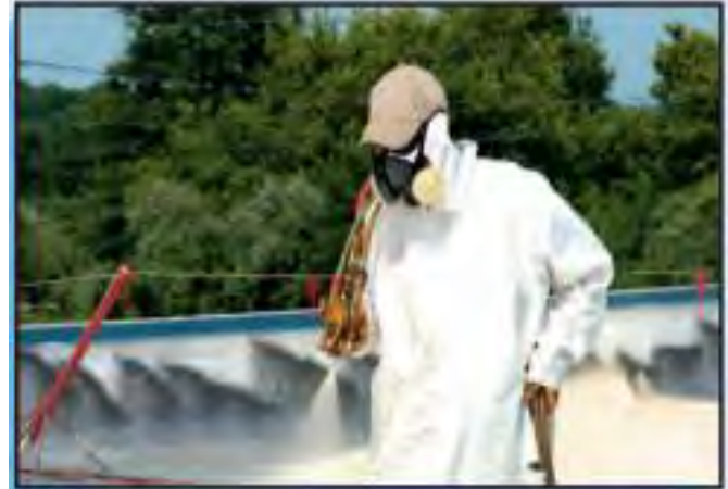
Worker applying SPF roofing material
