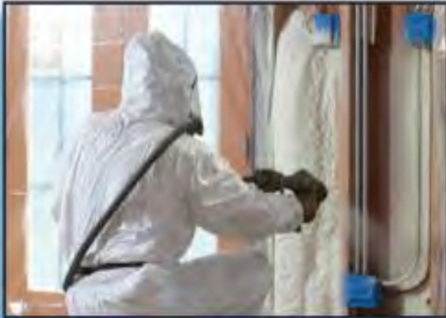
Worker applying SPF interior insulation
